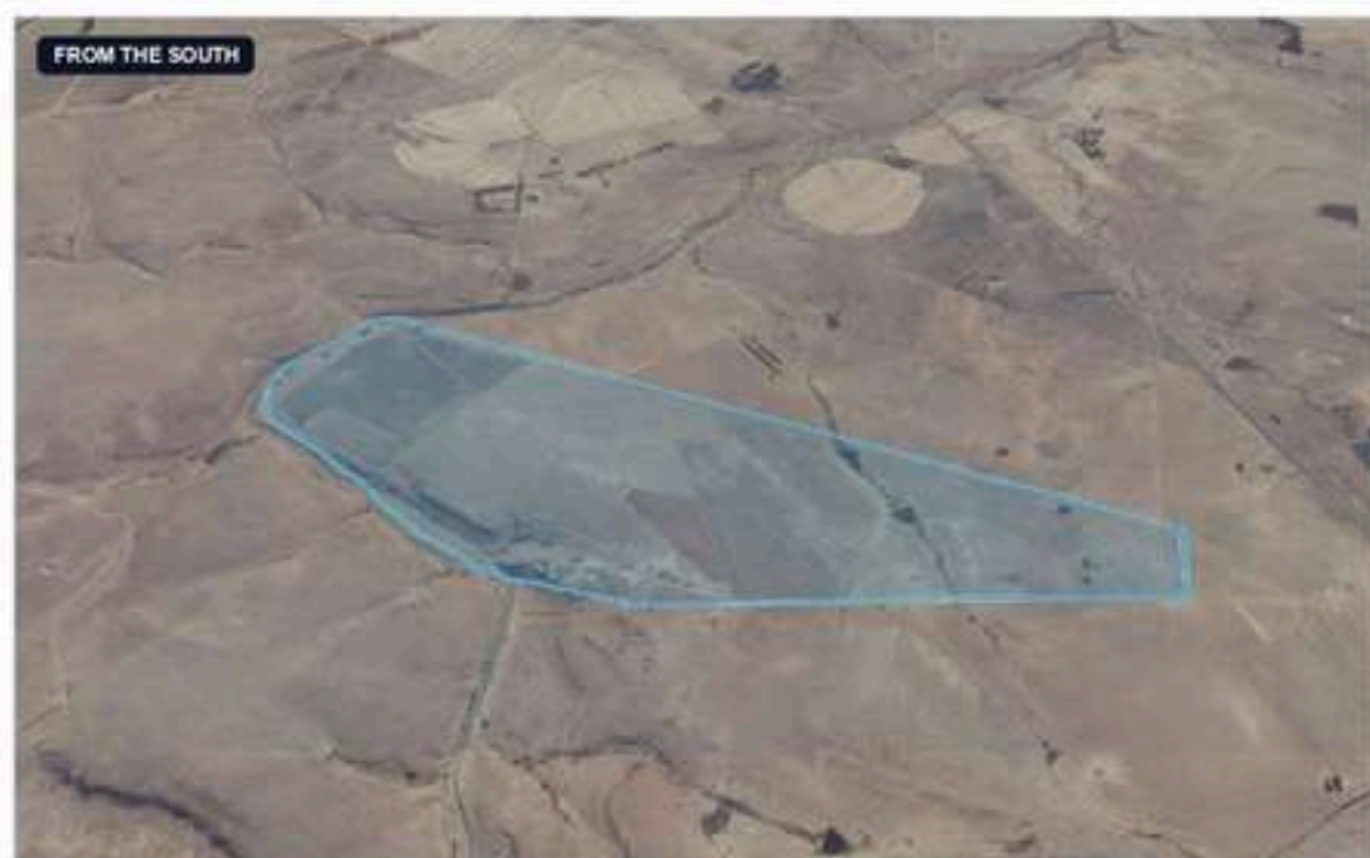
View from the south
