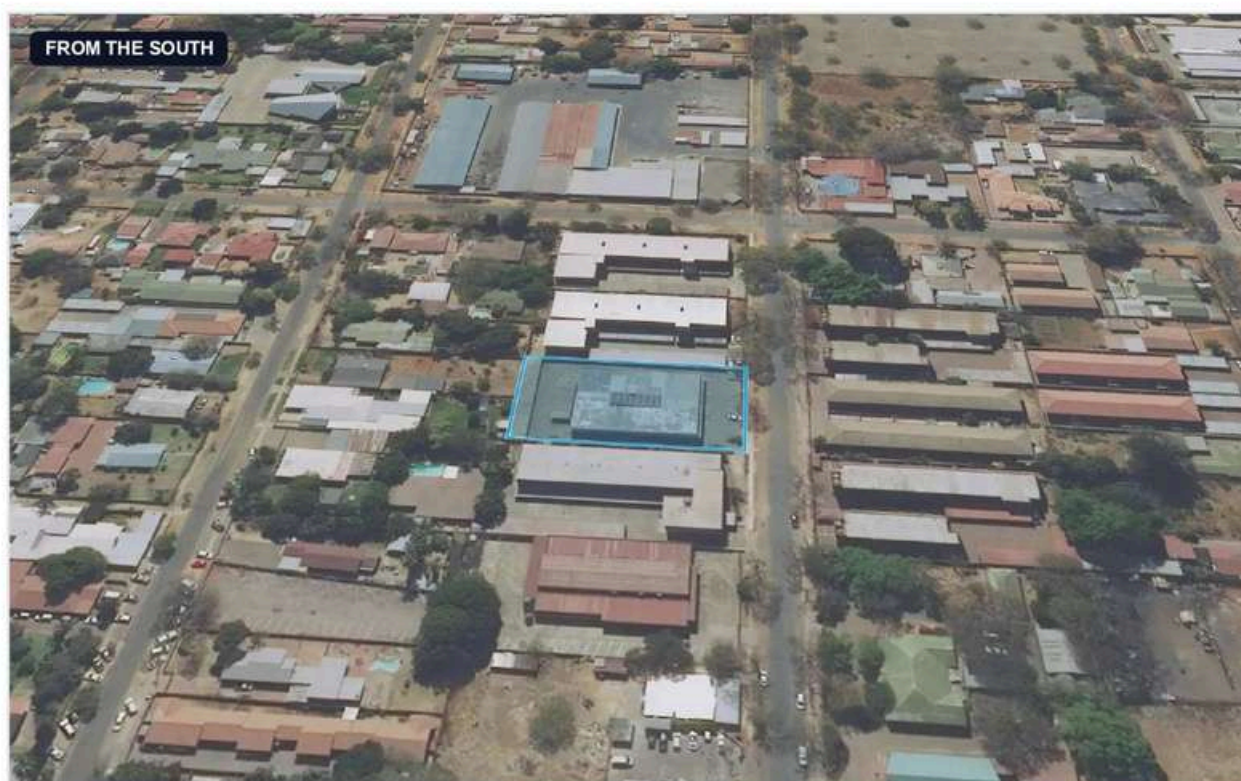
View from the south
